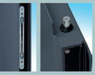
The inactive leaf is secured with flush bolts to the top and bottom of the leaf.
